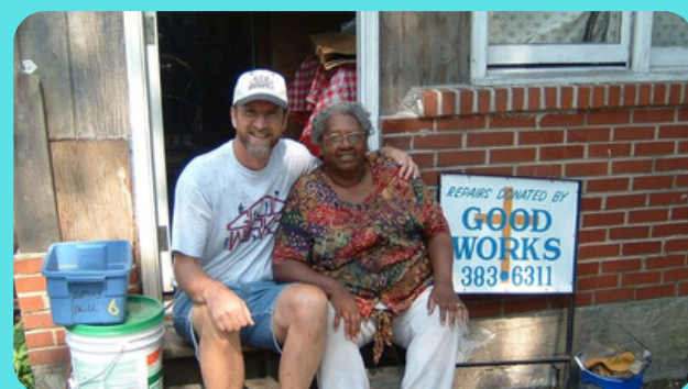
Good works helping a Phoenixville homeowner.
